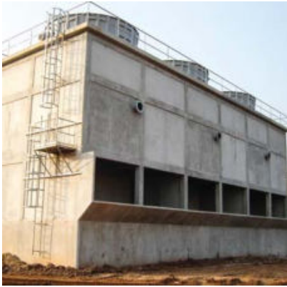
Sricharoen Biomass Power Plant, Burirum
